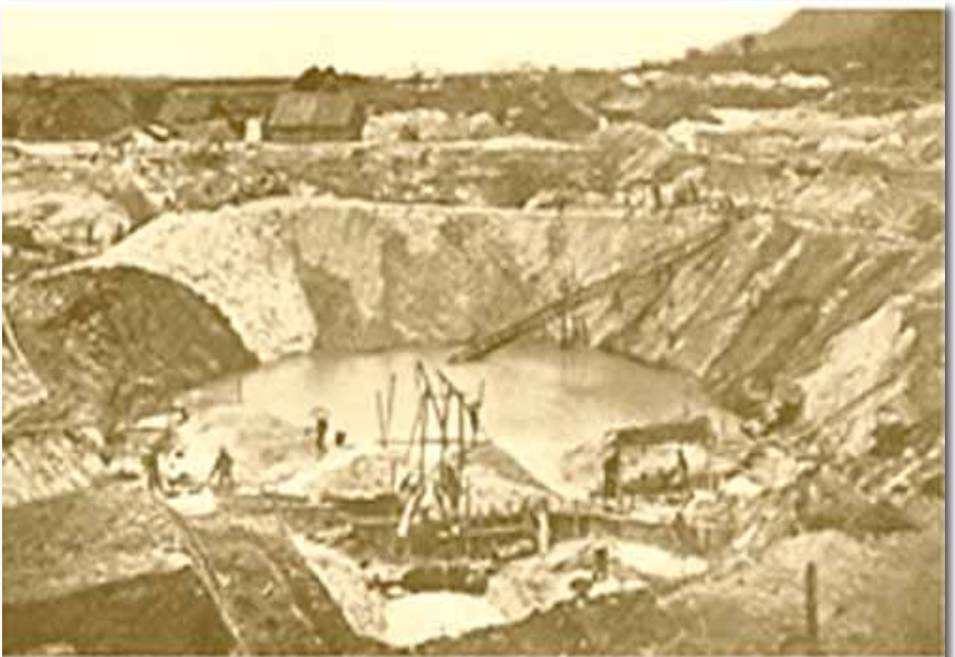
An open pit tin mine which is how Sunway Resort must have looked many years before
